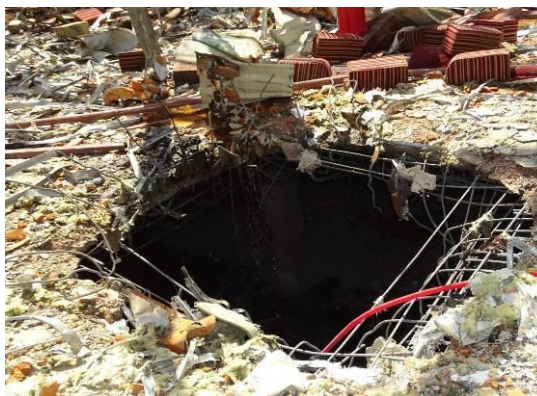
Figure 49.D.5 Entry point EO 2
