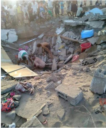
Figure 49.B.2 Civilian house post-explosion 243
