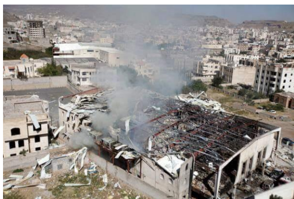
Figure 49.D.2 Post blast aerial image 298
