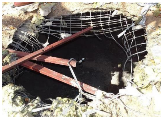
Figure 49.D.4 Entry point EO1
